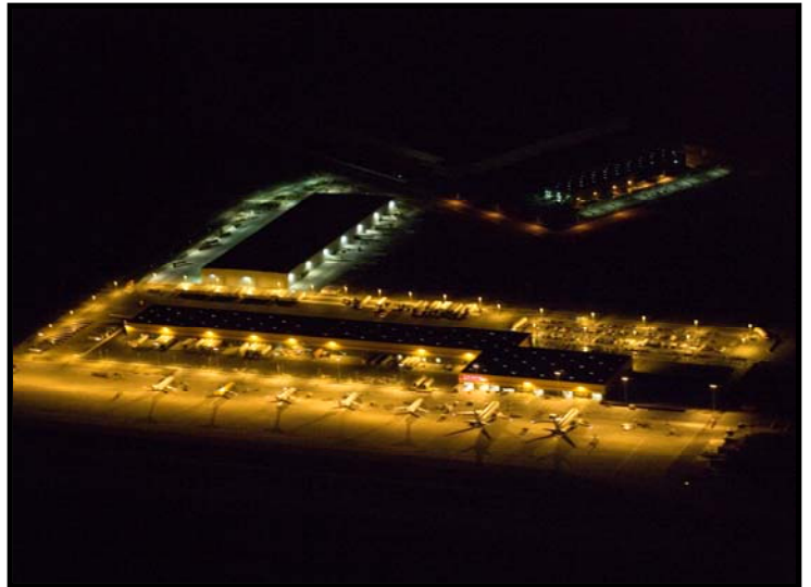
Airport /Airport Buildings and more
